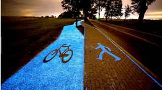
Figure 68 Glow in the dark surface treatment applied to a walking and cycling path
