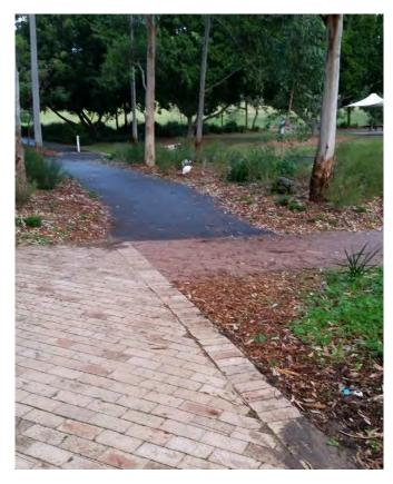
Figure 42 Undesirable dog-leg in the shared path
